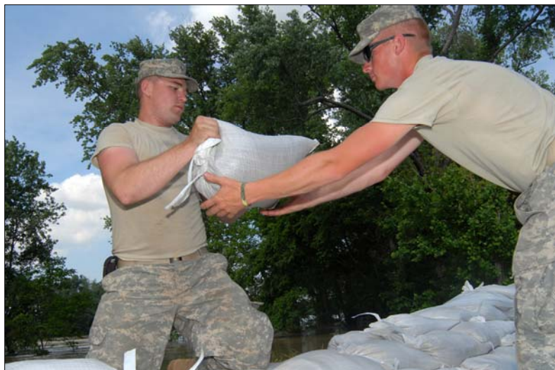
Members of the Indiana Army National Guard lay sandbags to prevent flood damage in Hazelton, Indiana.
